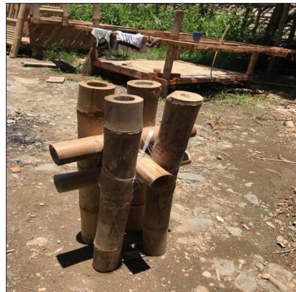
Fig. 4. Column and Beam Connection.
