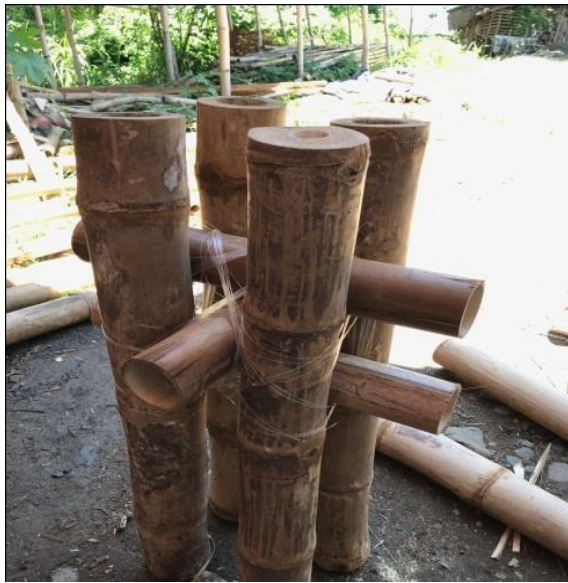
Fig. 5. Column and Roof Connection.
